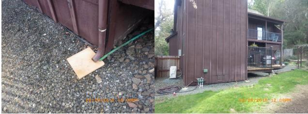
Avoid any wood soil contact, 4 inch clearance recommended. Various support posts were installed with steel deck screws.
