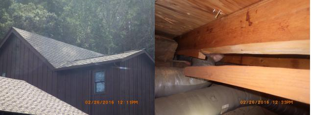
No visible sign of deflection in the roof from the exterior, attic interior shows one damaged rafter that should be repaired.
